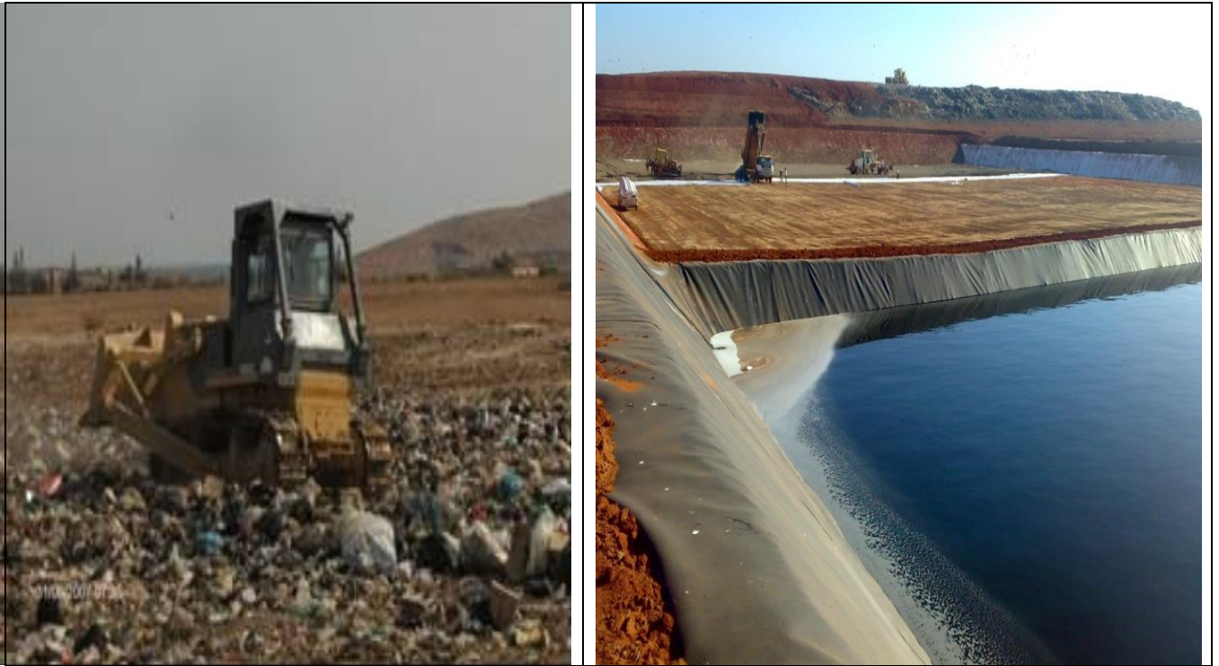
Figure 3: Leachate storage pond at the Oum Azza landfill.
