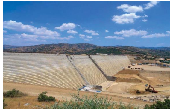
Fig. 8. Downstream face of Beydag dam
