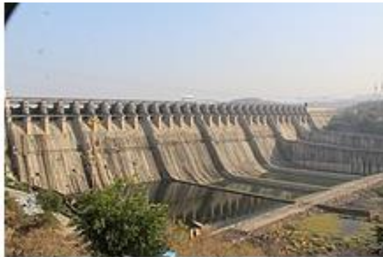
Fig. 1. Mass concrete structure of Sardar Sarovar Dam on Narmada River
