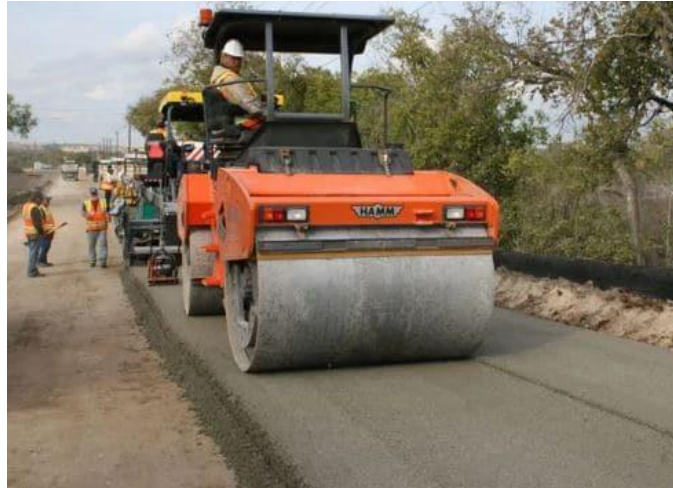
Fig. 6. Roller Compacted Concrete for Road Construction
